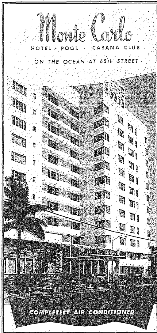
Figure 27 In 1951, a major addition was built on the south side (right) of the Monte Carlo Hotel. It was designed by the principal architect Albert Anis and the associate architect Melvin Grossman in the Post War Modern style. The 44-room, southern addition incorporated a portico that floated over the entrance (now altered, see also Figure 4), stone-faced wall panels and ribbon windows on the ground floor, corner windows on the upper floors, and a commanding group of decorative square vents at its crescendo.
