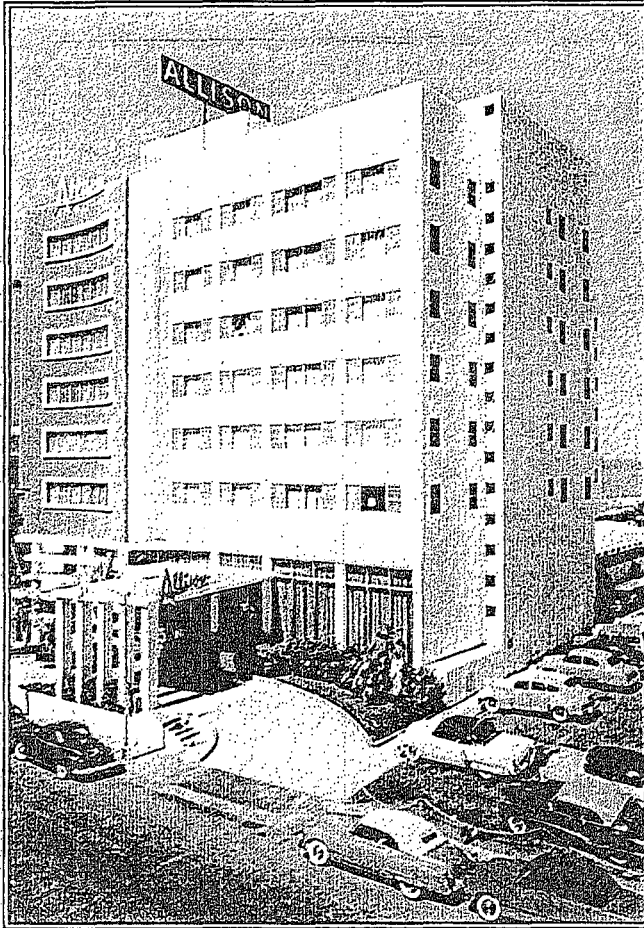
Figure 32 The Allison Hotel (now the Comfort Inn) was constructed at 6261 Collins Avenue in 1951. It was designed by A. Herbert Mathes in the Post War Modern style. The front elevation of the hotel featured a fabulous projecting concave wall with a fluted stucco finish and boxed ribbon windows. This curved wall was supported by columns with floating planes. The hotel's front elevation also maintained a dramatic porte-cochere and neon signage in the spirit of the post war automotive age.
